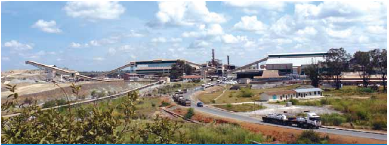
Panorama of Chambishi Copper Mine processing plant
