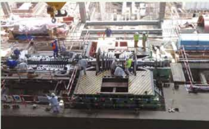
An aerial view of unit-1 turbine works
