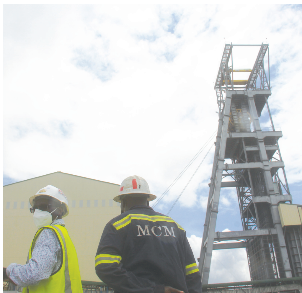
THE Synclinorium Shaft was launched in 2016 to reach a new ore body.
